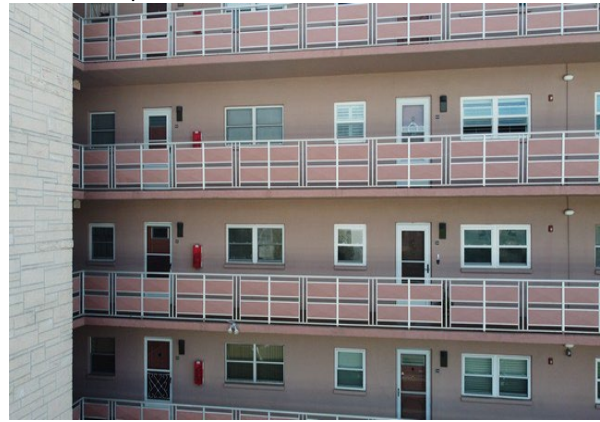
52 Front of Building
