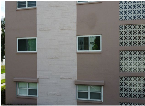
51 Front of Building
