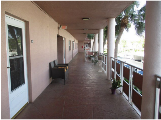
41 2nd Floor Walkway
