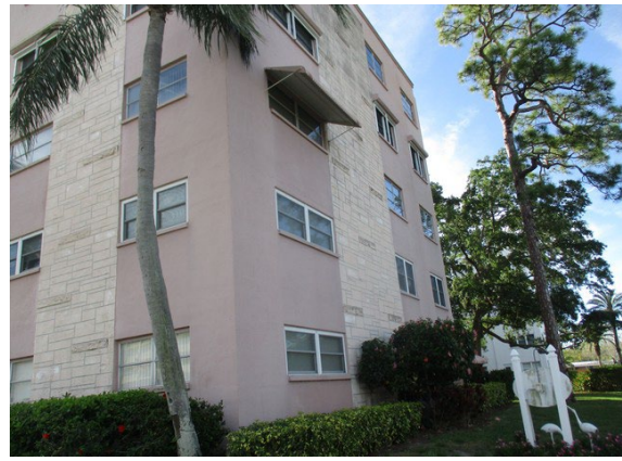
2 Right Side of Building
