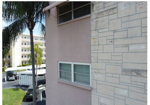
56 Right Side of Building
