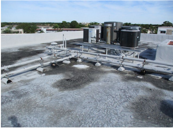
11 Roof Overview & HVAC Stands
