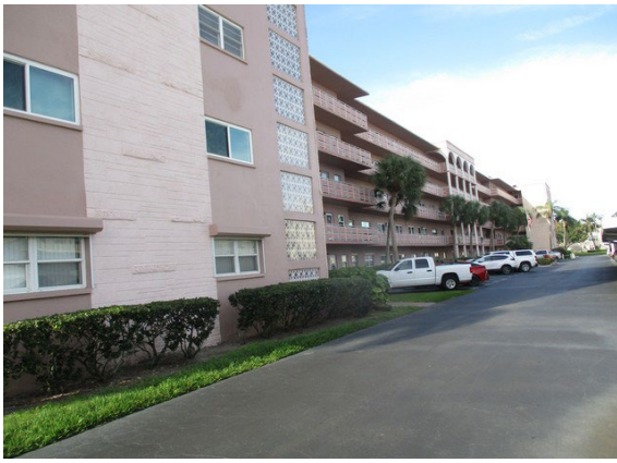
1 Front of Building
