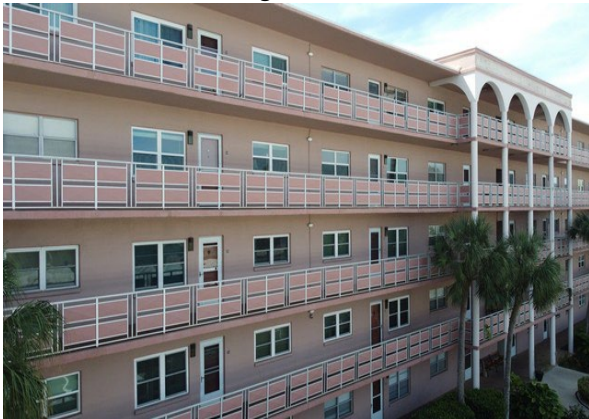
53 Front of Building
