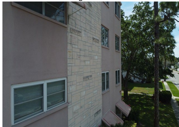
55 Right Side of Building
