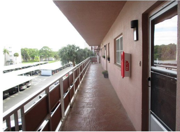
36 3rd Floor Walkway
