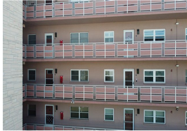
52 Front of Building
