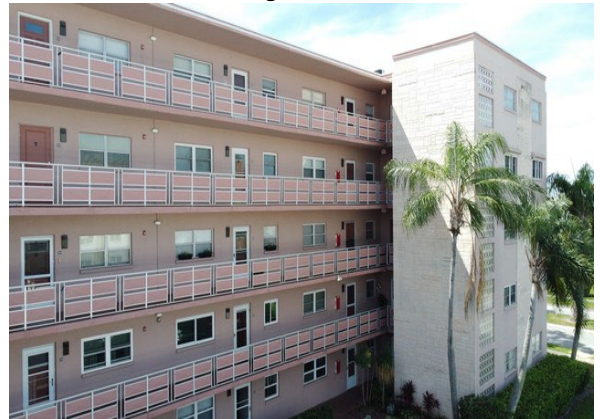
54 Front of Building
