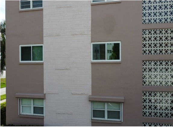
51 Front of Building
