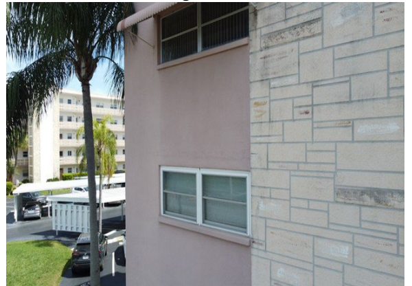
56 Right Side of Building
