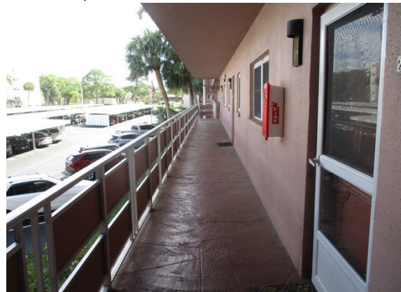
40 2nd Floor Walkway
