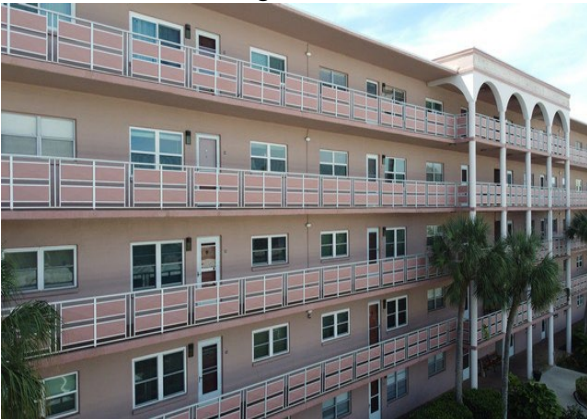
53 Front of Building
