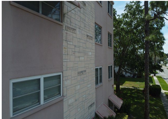
55 Right Side of Building
