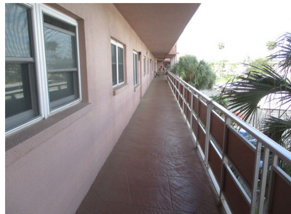
37 3rd Floor Walkway
