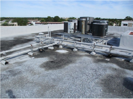
11 Roof Overview & HVAC Stands
