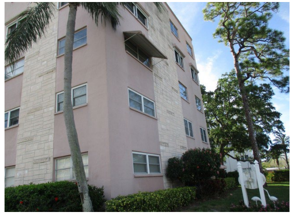
2 Right Side of Building
